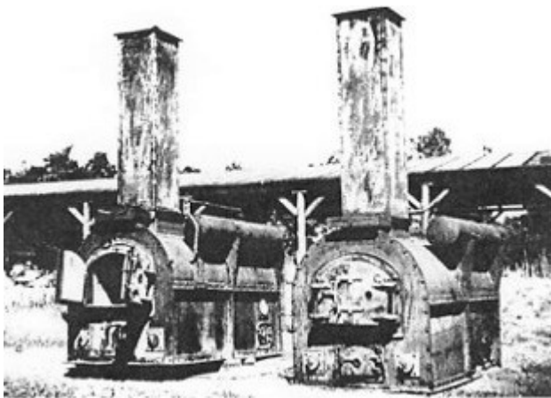
Illustration 4: The two transportable field crematoria (when they were in operation the height of the chimney was doubled by adding a second segment). Source: The film "Todeslager Sachsenhausen", DEFA 1946.
